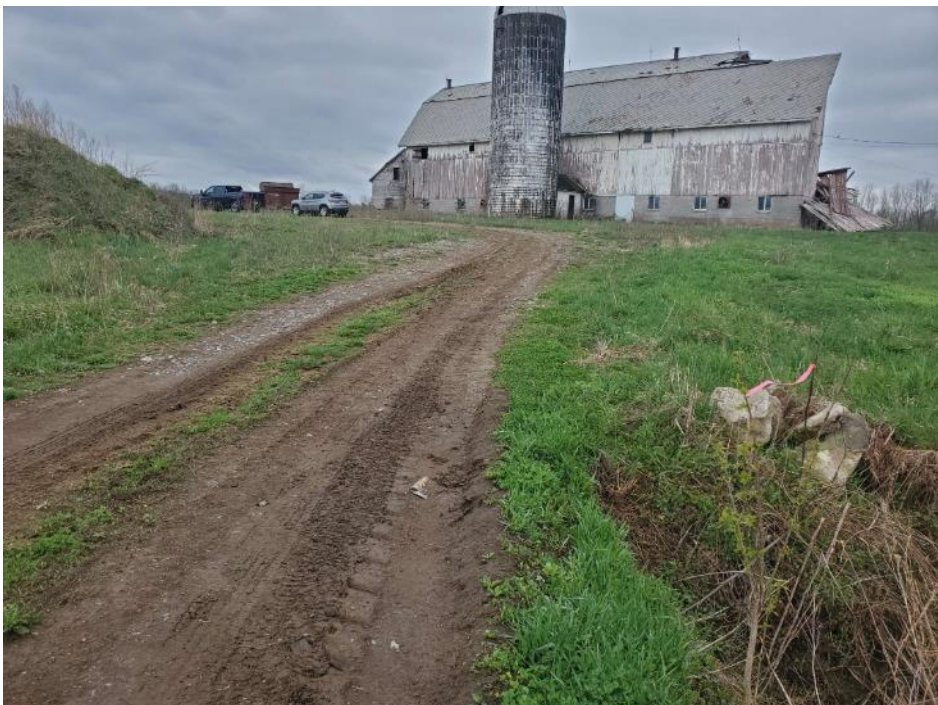
Photo 8 – Representative photo of the northwestern corner of the site.
