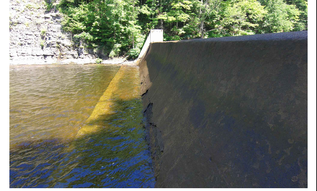
PHOTO 3 - SPILLWAY AND RIGHT NON-OVERFLOW SECTION
