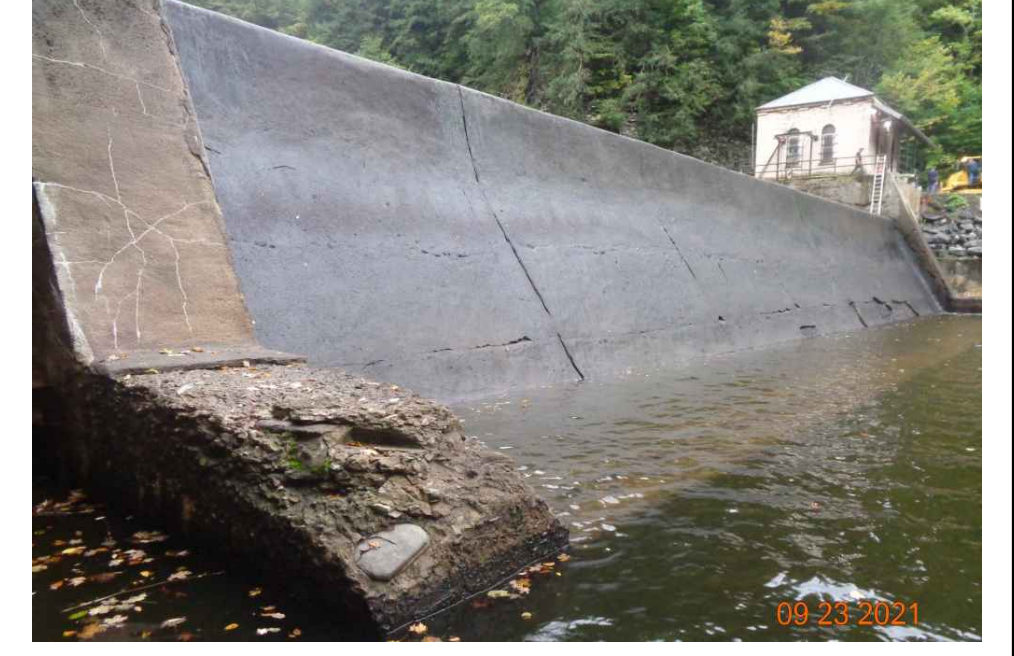
PHOTO 4 - RIGHT TRAINING WALL AND DOWNSTREAM FACE OF SPILLWAY
