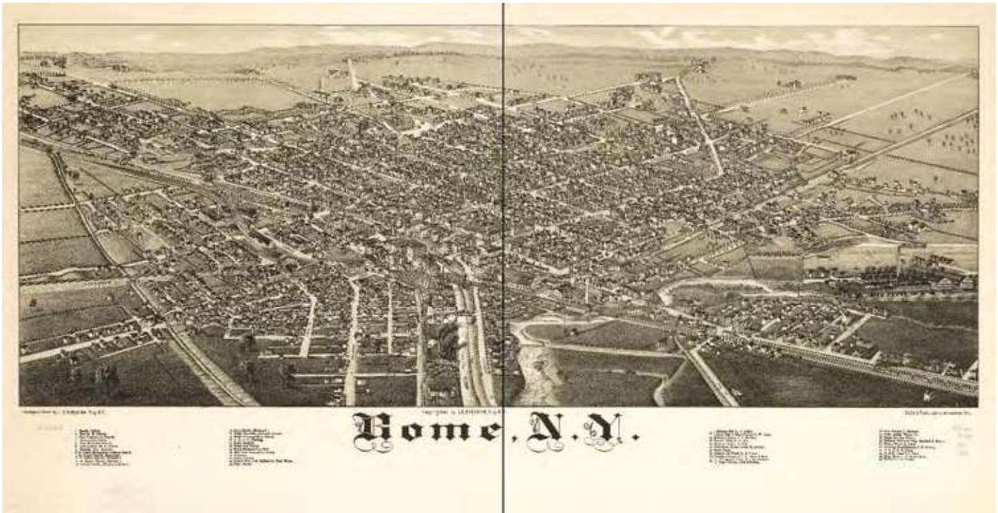
Figure 8. Rome had a dense downtown and robust infrastructure in this 1886 birds-eye view. Some district properties that are easily distinguishable in this view include the cemetery (now Fort Stanwix Park), where the diagonal Turin Street meets James Street; almost kitty-corner from the cemetery is the John B. Jervis House, which towers above the other houses around it. Library of Congress, available online at https://www.loc.gov/item/75694841/ .
