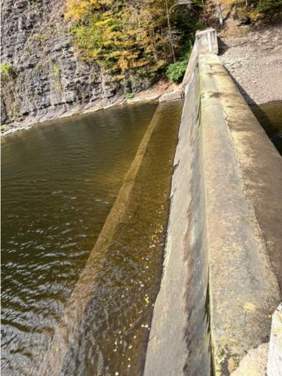
Oct. 2024 – reservoir drained for work in lower level of gatehouse
