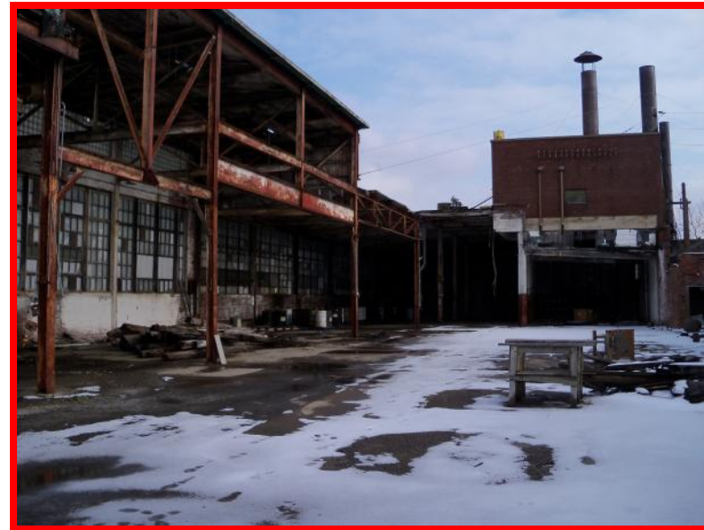
Photo 5 Building # 1 2004 Corrosion of frame and roof decking. Some bricks have fallen from under the window.
