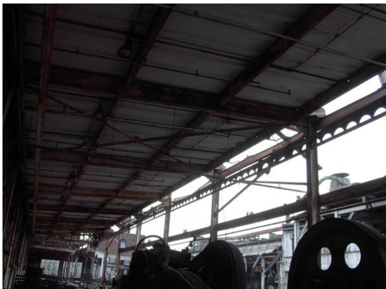
Photo 4 Building # 1 Corrosion of roof decking.
