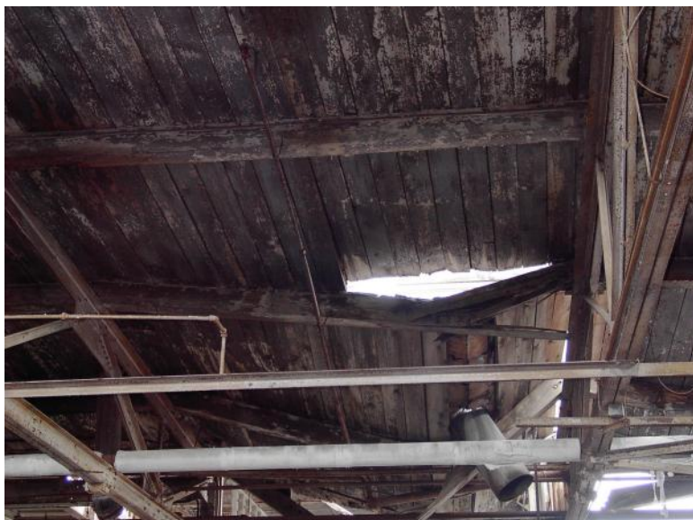
Photo 37 Building # 6 2004 More of the wood roof deck is collapsing
