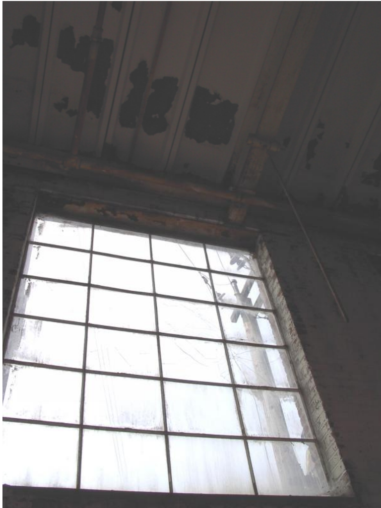
Photo 11 Building # 1 2004 Ongoing corrosion of roof decking.
