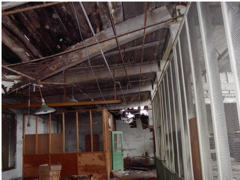
Photo 48 Building # 4 2004 Area no longer safe so angles and location do not match – new photo shows partial roof collapse.
