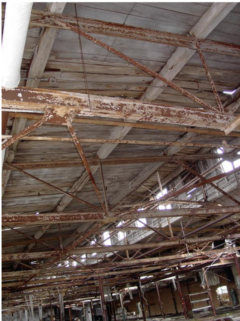
Photo 34 Building # 6 2004 More of the wood roof deck is collapsing.
