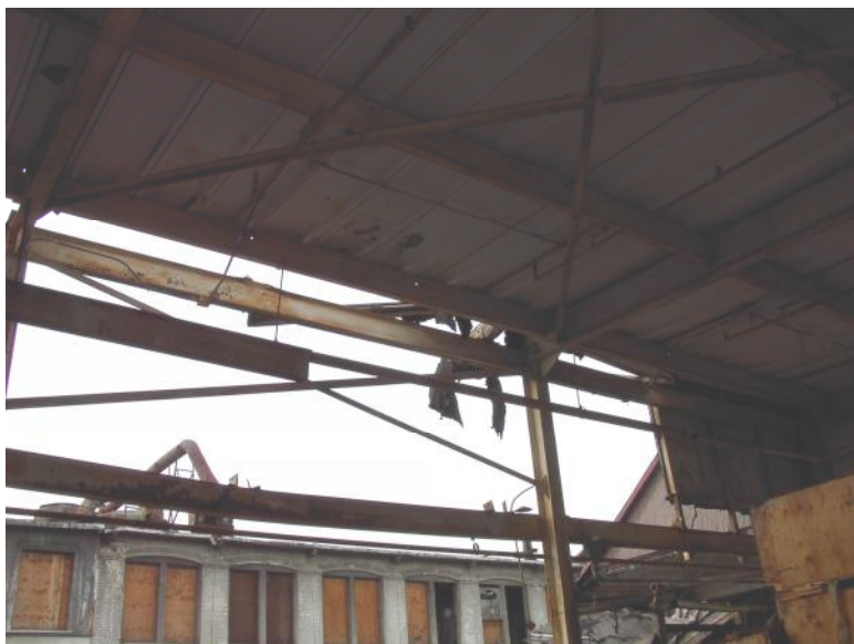
Photo 3 Building # 1 Some loose roofing materials have fallen.
