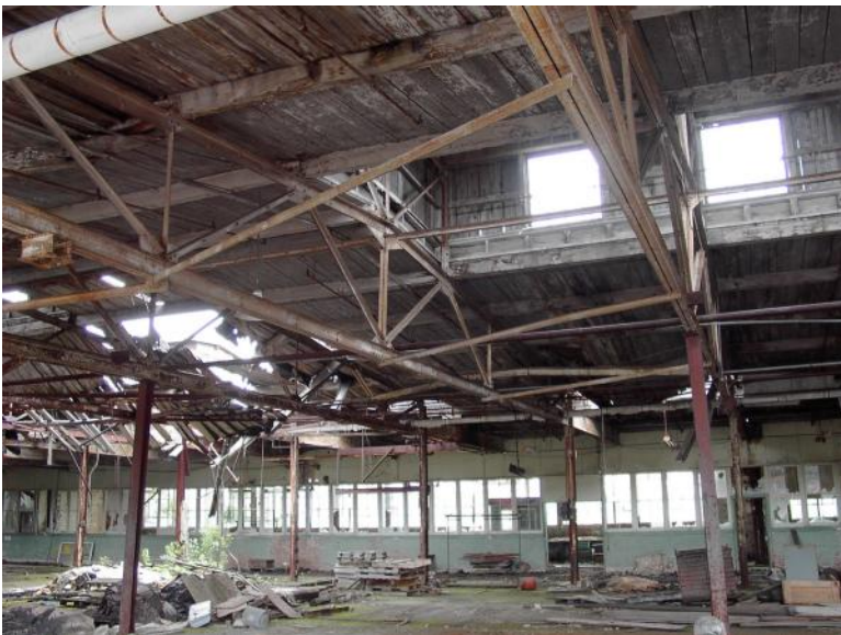
Photo 32 Building # 6 More of the wood roof deck is collapsing.
