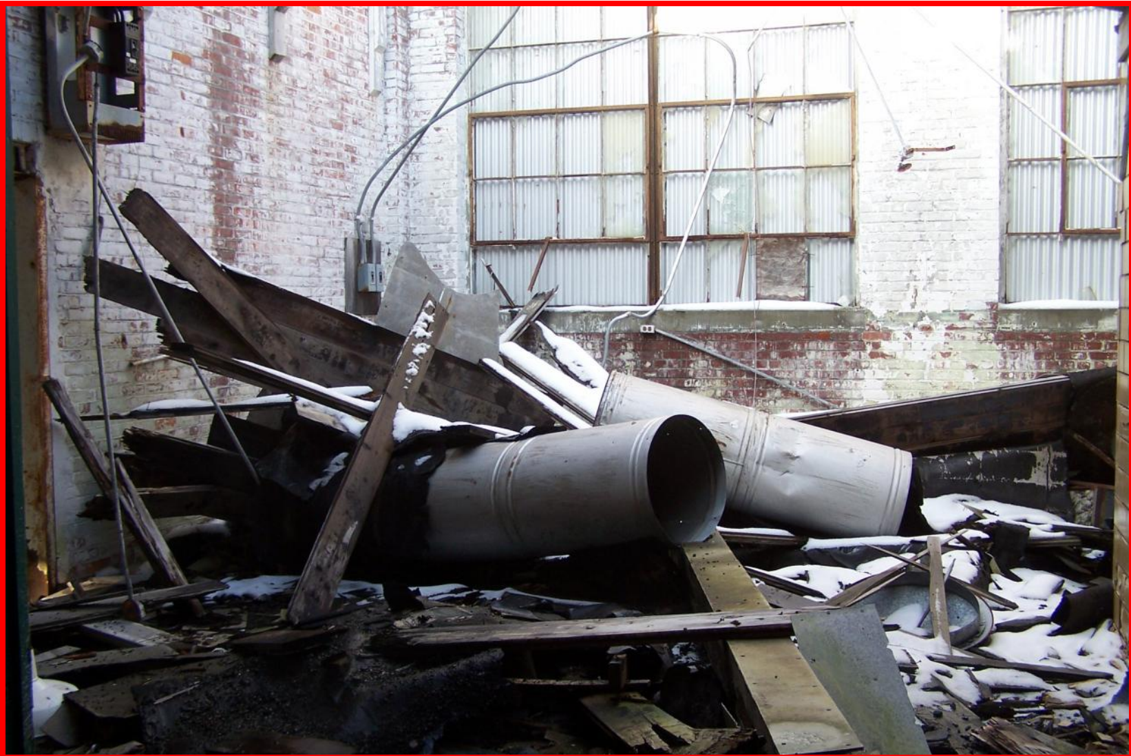
Photo 58 Building # 6 Significant collapse including a tall chimney or vent pipe
