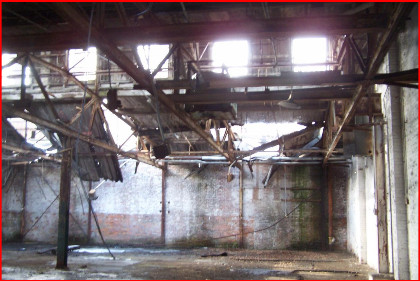
Photo 59 Building # 6 Significantly more of the wood roof deck is collapsing.
