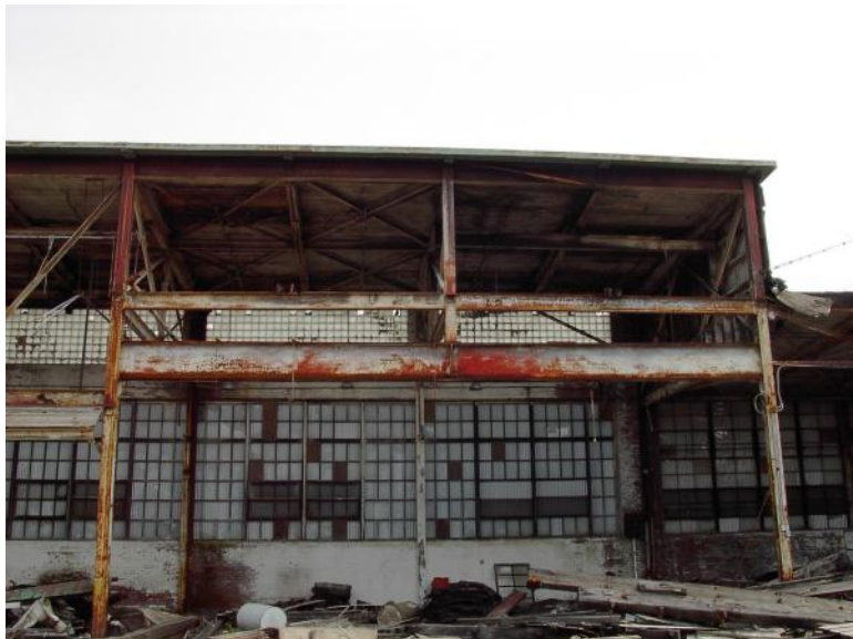
Photo 10 Building # 1 2004 Debris has been removed. New holes in the roof decking.
