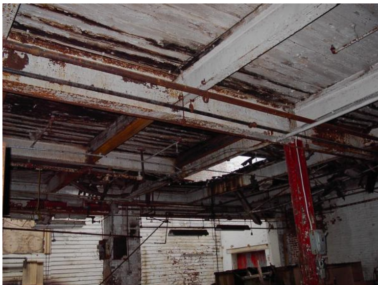
Photo 45 Building # 3 / 4 (Downstairs) 2004 More of the floor is collapsing
