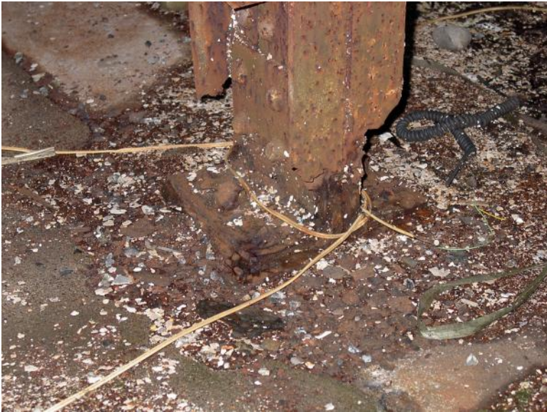
Photo 24 Building # 6 Corroded column base not repaired
