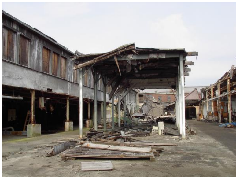
Photo 7 Building # 1 / 2 2004 Debris has been removed. Wooden roof members have shifted and fallen.
