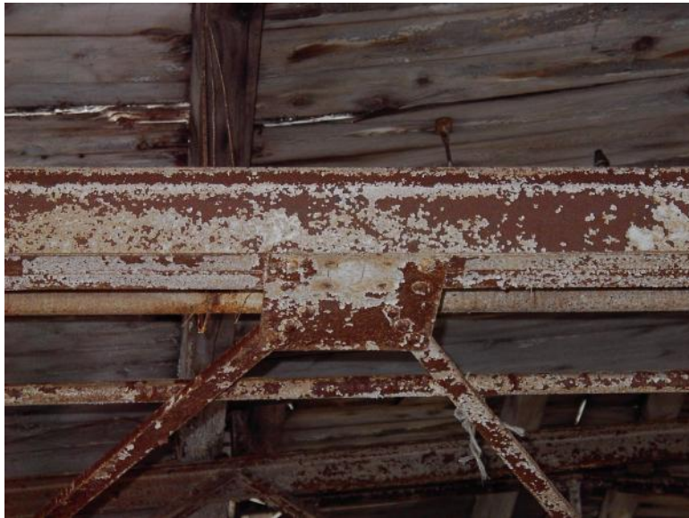
Photo 35 Building # 6 2004 More of the wood roof deck is collapsing.
