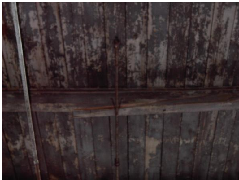
Photo38 Building # 6 2004 More of the wood roof deck is collapsing
