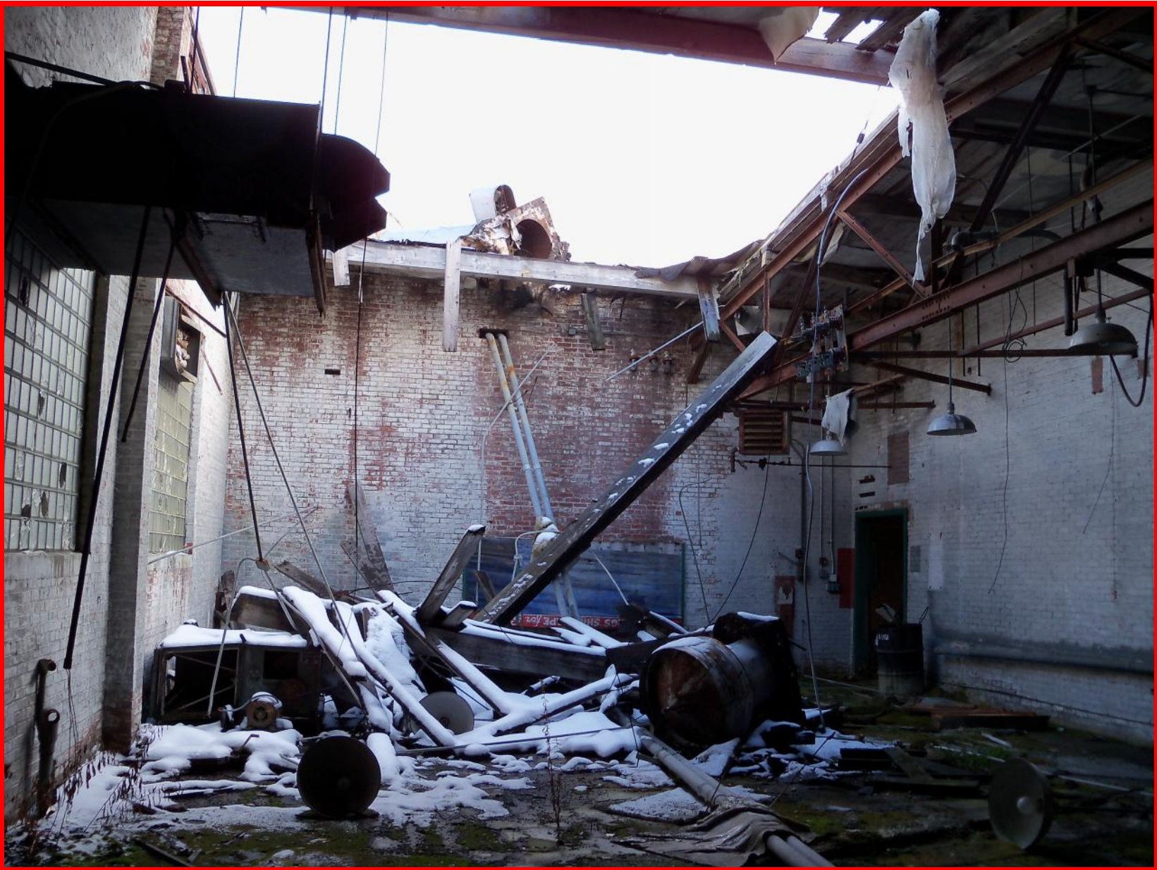
Photo 57 Building # 6A Significant collapse including a tall chimney or vent pipe
