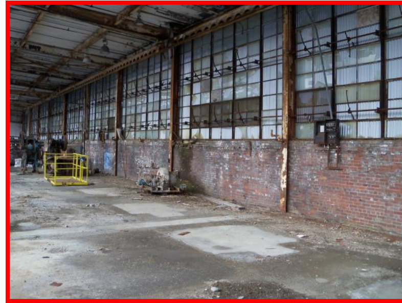
Photo 5 Building # 1 2004 Corrosion of frame and roof decking. Some bricks have fallen from under the window.
