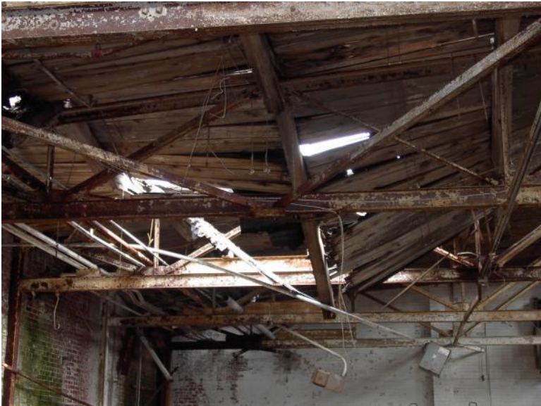
Photo 22 Building # 6 2004 More of the wood roof deck is collapsing
