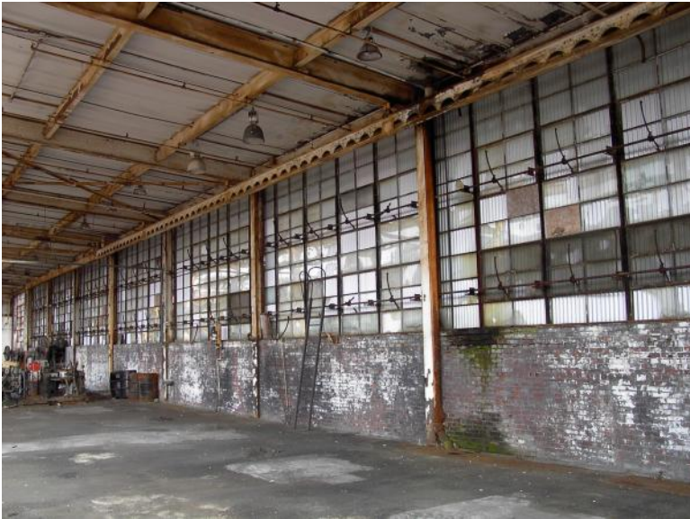
Photo 5 Building # 1 2004 Corrosion of frame and roof decking. Some bricks have fallen from under the window.
