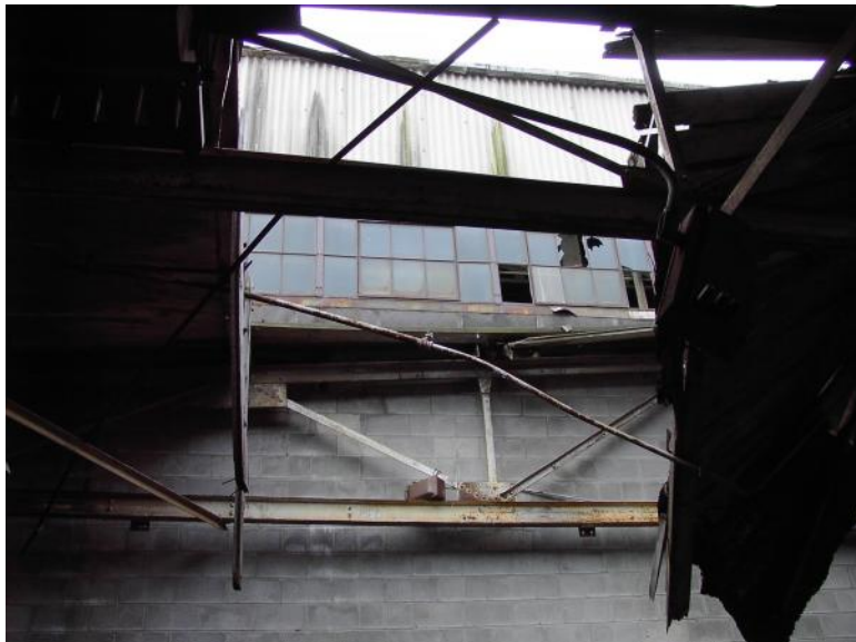
Photo 27 Building # 6 (39 High-Bay Beyond) 2004 More of the wood roof deck is collapsing
