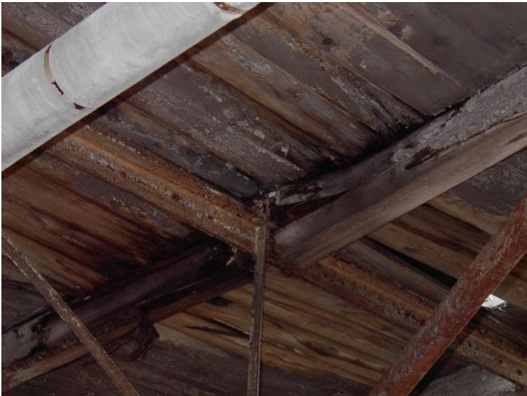
Photo 21 Building # 6 2004 More of the wood roof deck is collapsing.
