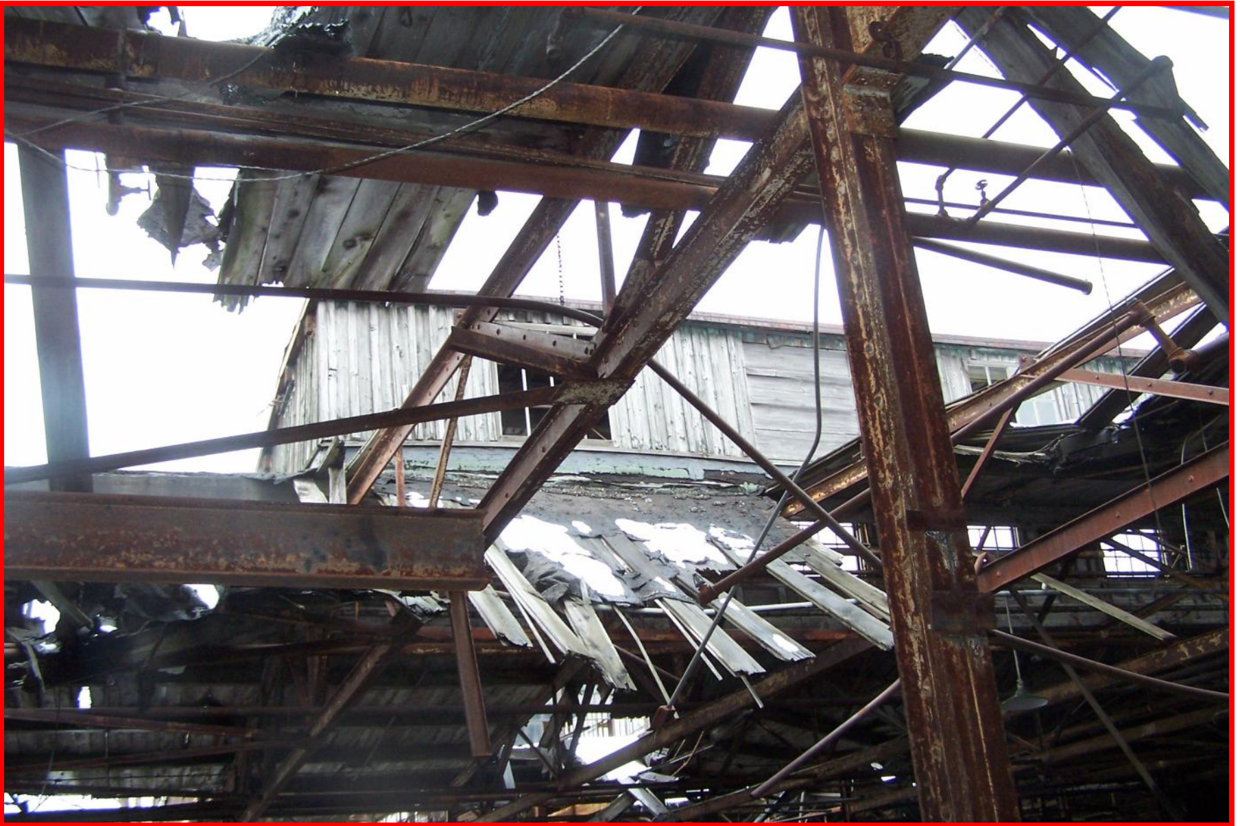
Photo 60 Building # 6 Significantly more of the wood roof deck is collapsing.
