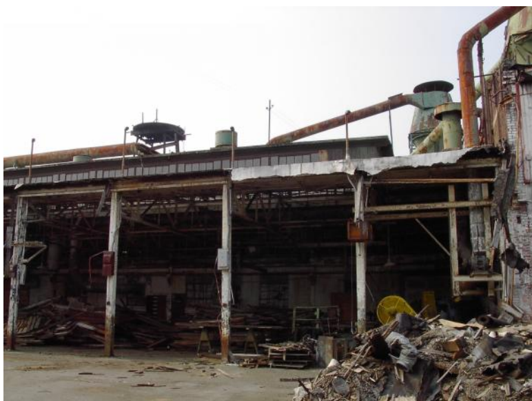
Photo 8 Building # 1 / 2 & 3 2004 Debris has been removed. Additional debris is piled.
