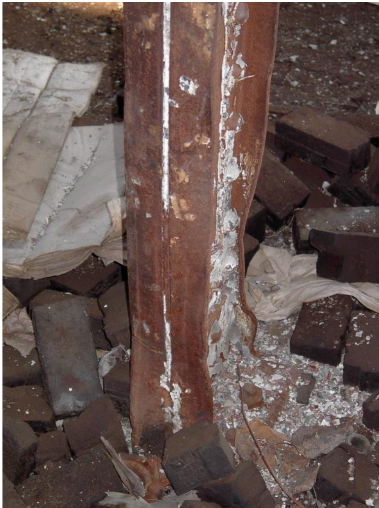
Photo 20 Building # 35 2004 Some debris removed. Distorted column base not repaired.
