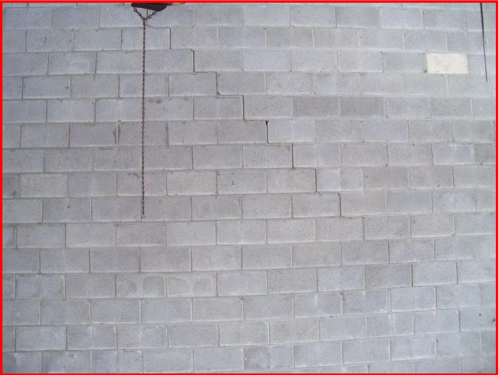
Photo 61 Building # 6 (39 High-Bay Beyond) 2004 Cracked masonry
