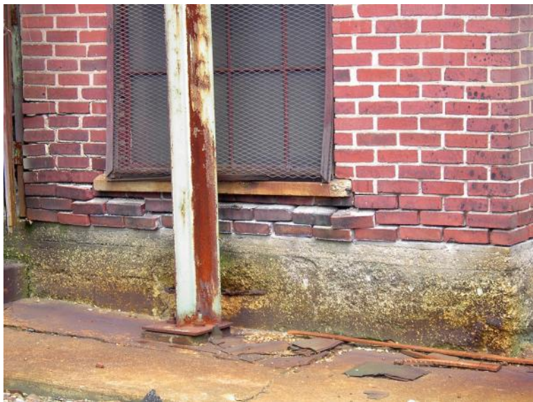
Photo 42 Building # 2A 2004 Loose bricks under the window not repaired.
