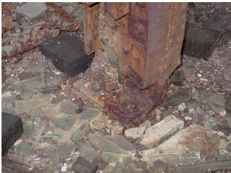
Photo 39 Building # 6 Corroded column base not repaired.
